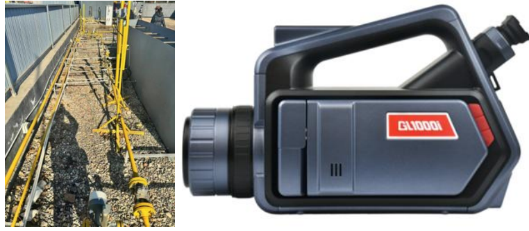
Figure 2. Hydrogen-blended Natural Gas Pipeline Leakage Pilot Area
