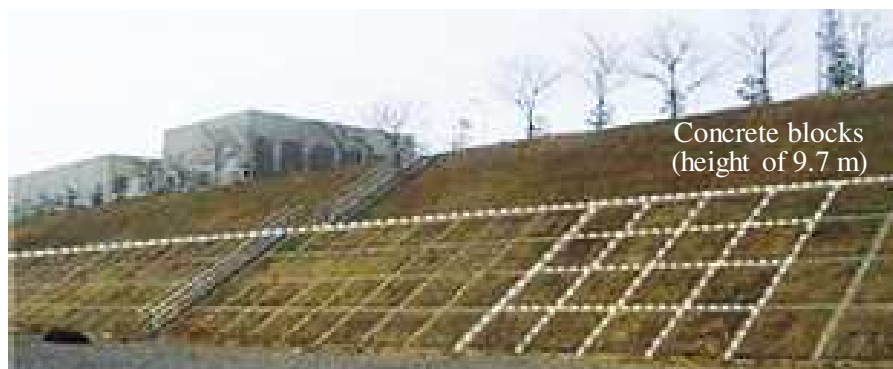
Figure 1. Construction status of concrete blocks.
