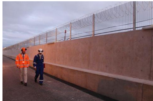
Figure 2 New Flood Wall
