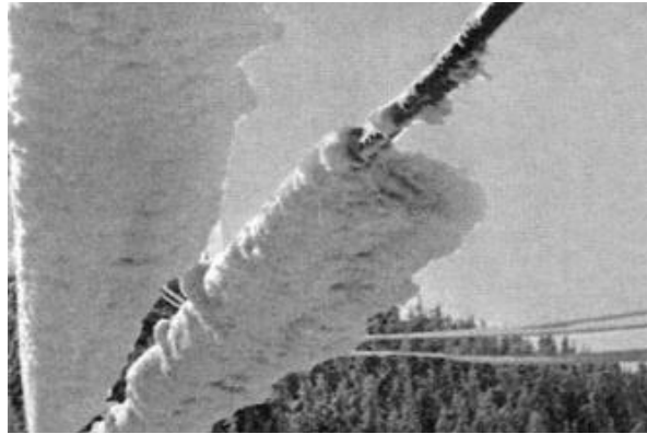
Figure 3: Conductor with ice formed in an incloud icing process
